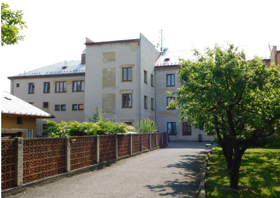
Budova D domova pro seniory
